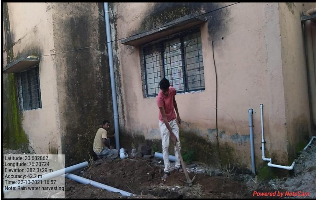
**PVC Pipes System for Roof Top Water Harvesting from Ladies Hostel**
