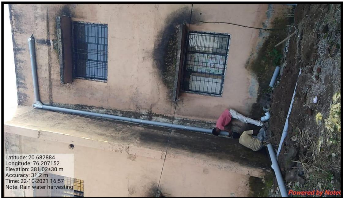
**PVC Pipes System for Roof Top Water Harvesting from Ladies Hostel**
